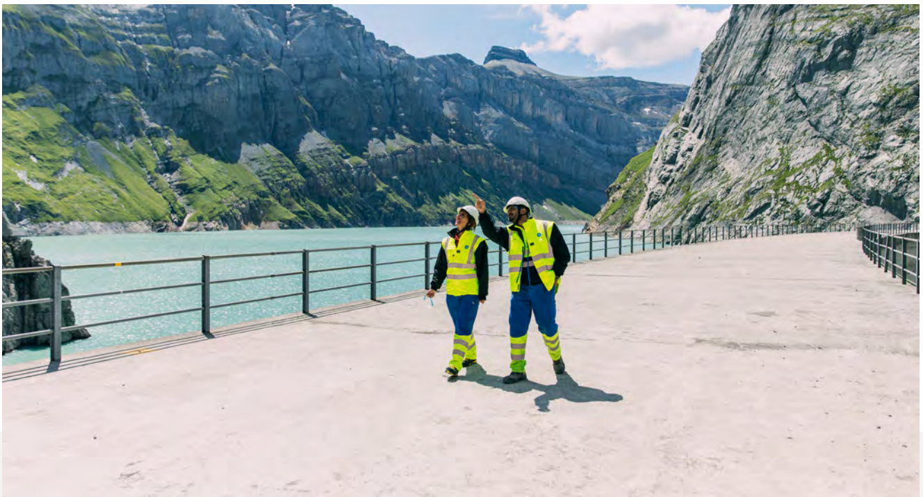
Hydro power stations, Linthal, Switzerland
