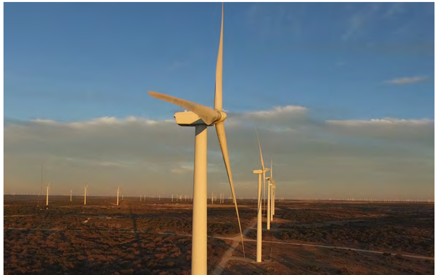
Wind farm in Texas, U.S.A.
